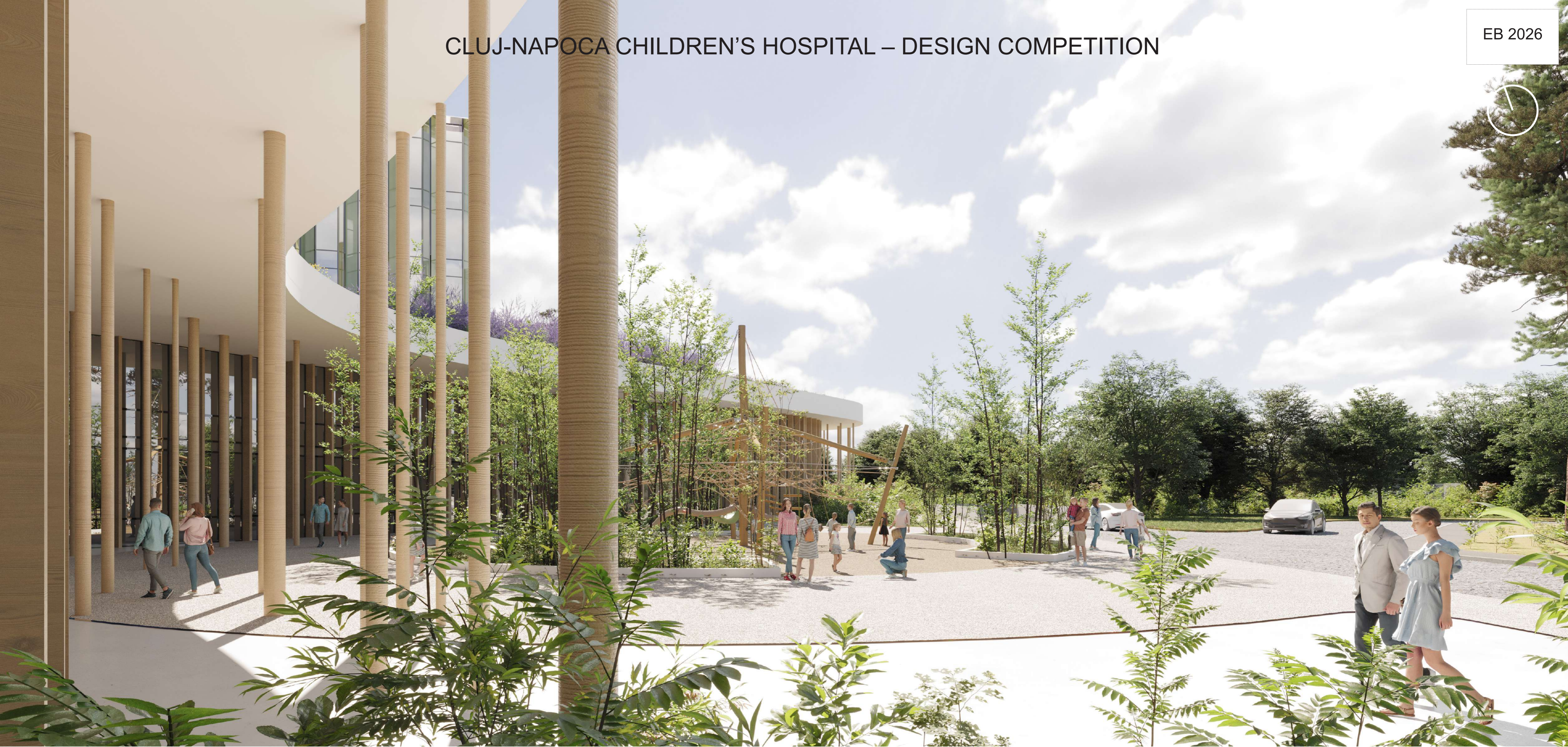
▲ VIEW OF THE "FOREST" OF WOODEN COLUMNS SUPPORTING THE OVERHANGING 3RD FLOOR ROOF GARDEN
